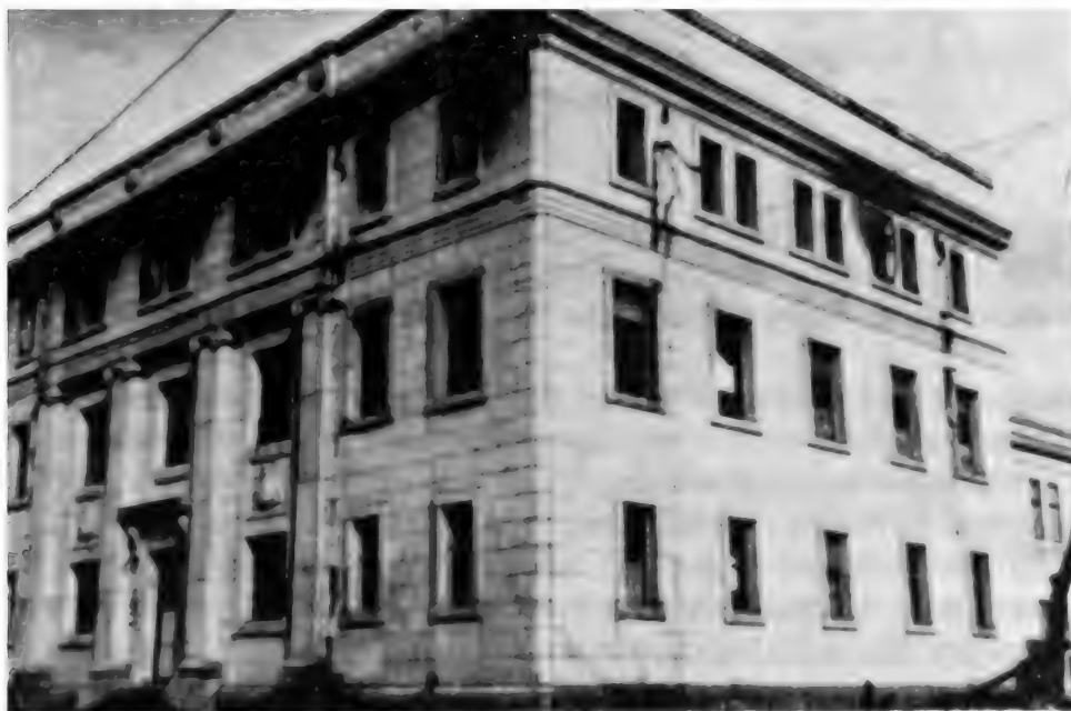
BANK OF JAPAN, HIROSHIMA (BUILDING 24)
